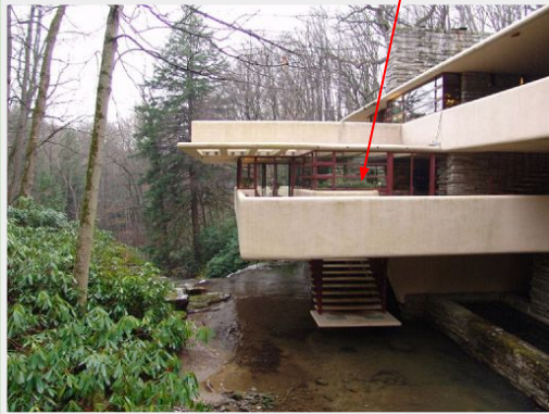
Frank Lloyd Wright / Fallingwater / 1964 / Architecture / 01-31-20 / http://www.wright-house.com/frank-lloyd-wright/fallingwater-pictures/7x-stairs-house-to-waterfall.html
